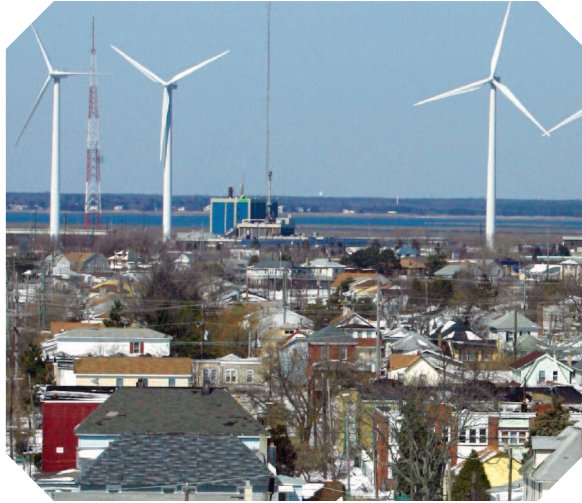
The Atlantic County Utilities Authority's wind energy project includes five 1.5 MW turbines visible from the Atlantic City Expressway.
